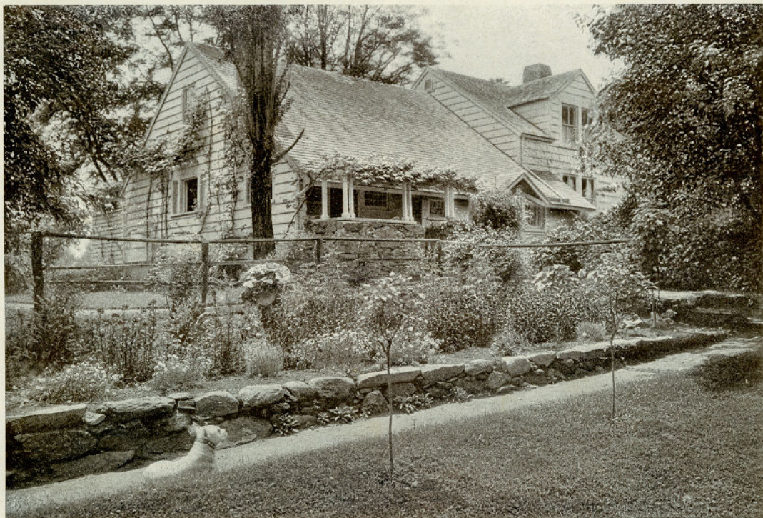
The dormer windows—an important element in the remodeling—relieve and animate the great expanse of roof
