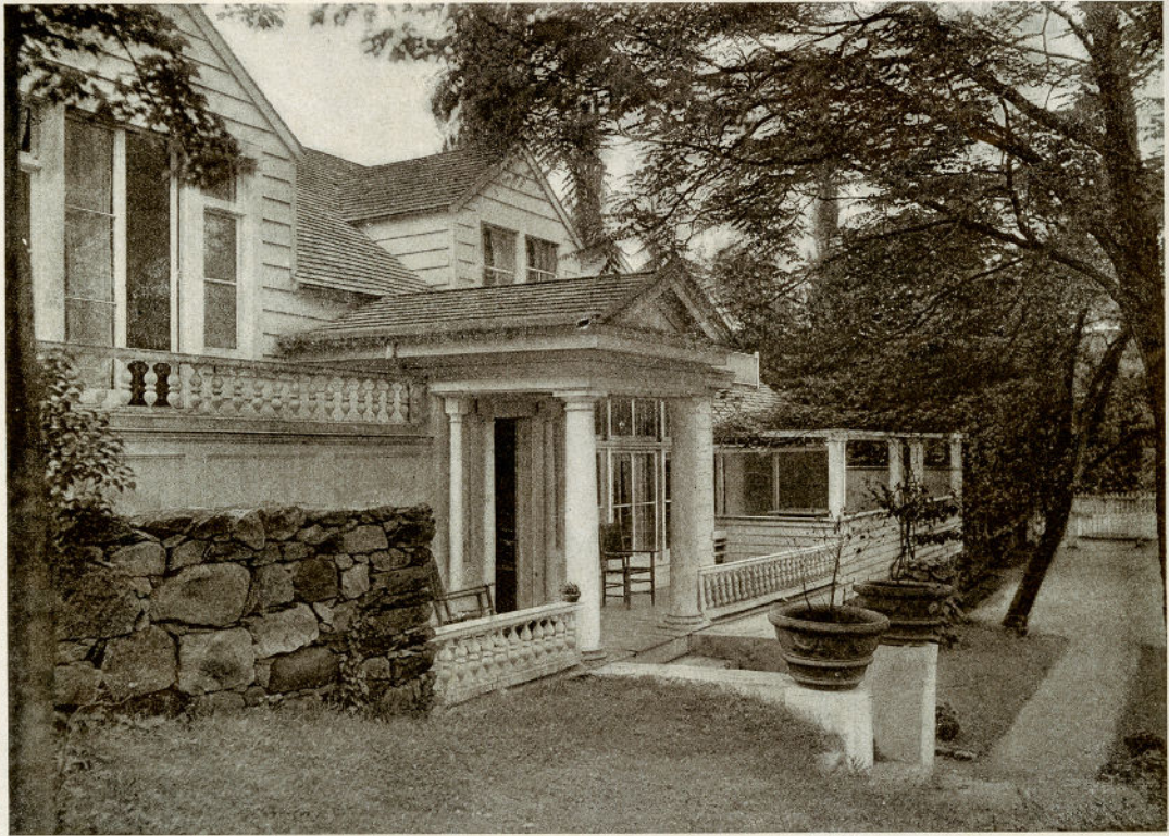
Fitting a house to a hill—the roof comes close to the ground at the west end of the second story
